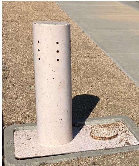
Figure 3. Typical Air Release/Air Vacuum Valve at Grade
